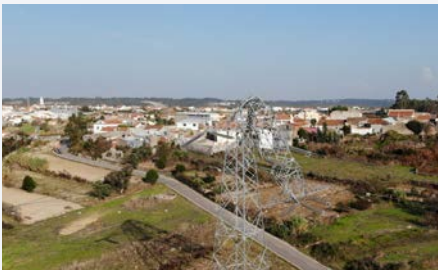
View of damaged trees and houses after Storm Leslie
