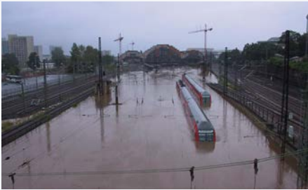
View of the flooded central train station by the River Weisseritz
