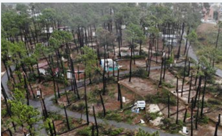
View of an electricity pylon bent by the winds of Storm Leslie
